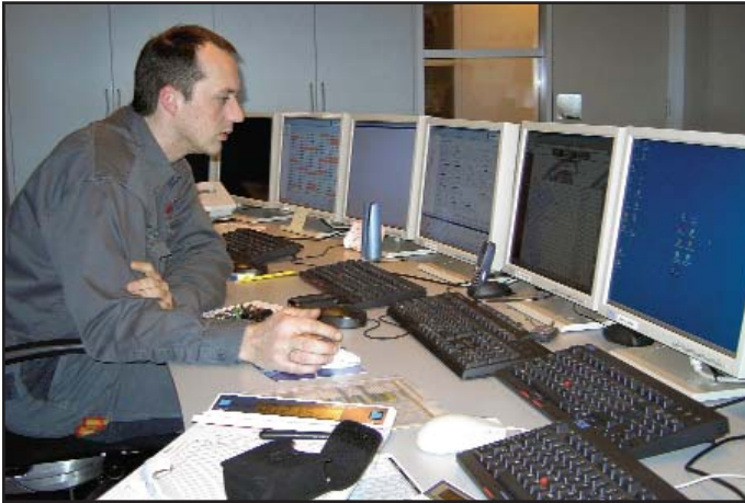
Elsam worker in Control Room
